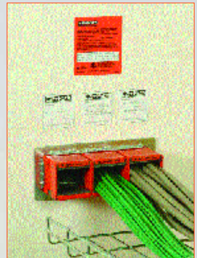
EZ-Path™ can be ganged for expansion or segregation of cables and provides excellent cable management.
