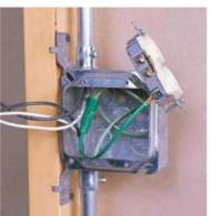
This connector is for connecting multiple grounding conductors to a device.
