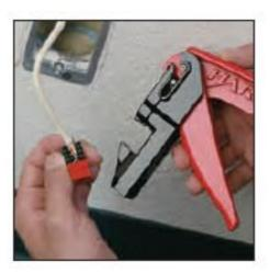
Release handle and remove jack from JackRapid tool. Visually verify proper termination.
