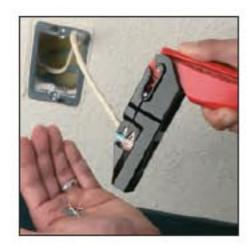
Wires will be seated and cut for a solid termination.
