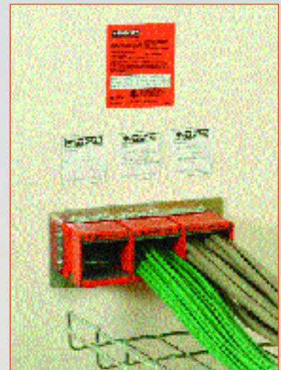
EZ-Path™ can be ganged for expansion or segregation of cables and provides excellent cable management.
