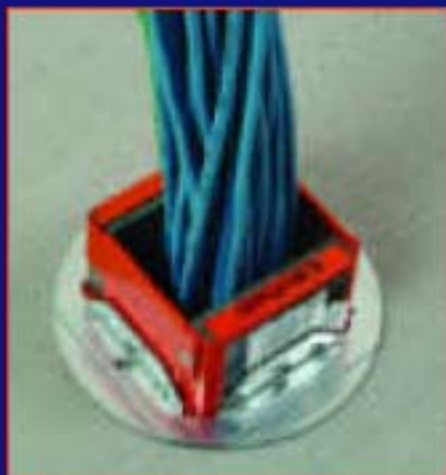
EZ-Path™ Floor Installation
