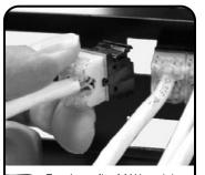
Terminate flat MAX modules and install into patch panel according to the instructions that accompanied the MAX modules.
