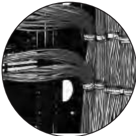
Unique fins support large bundles of cable
